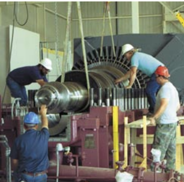
This 42 MW steam turbine generator set is being prepared for operation in a one-on-one combined cycle installation.
