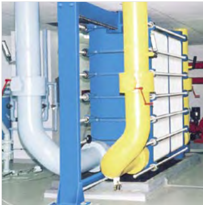
HVAC Thousands of SUPERCHANGER heat exchangers are in HVAC service for “free cooling” and isolation purposes. “Free cooling” payback is typically less than one year.
