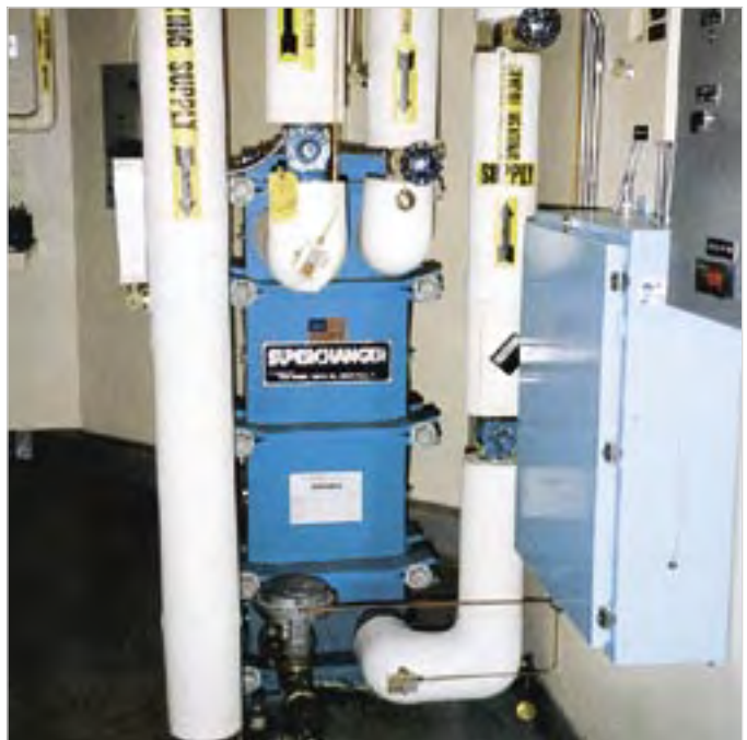
Waste Heat Recovery SUPERCHANGER heat exchangers recover heat very efficiently because of their high heat-transfer rates and close temperature approach capabilities.
